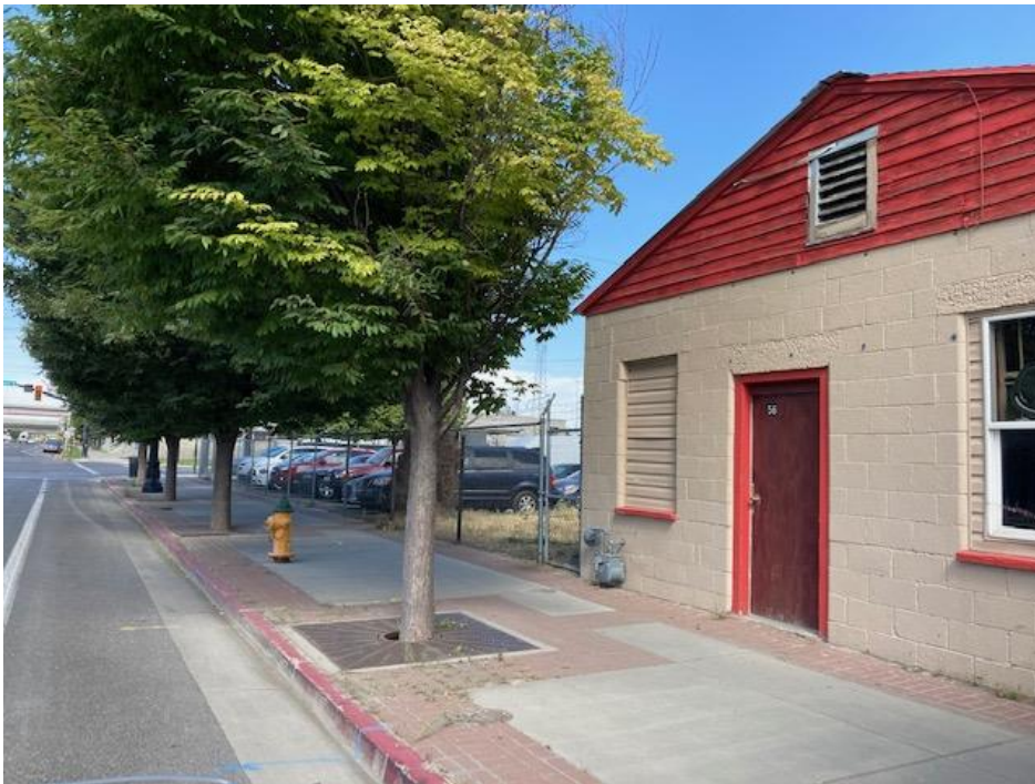
Street frontage along 200 S looking west.
